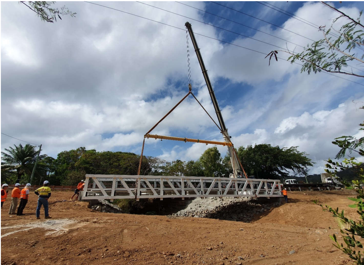
Cycle/Footpath at Two Mile Creek Bridge Construction
