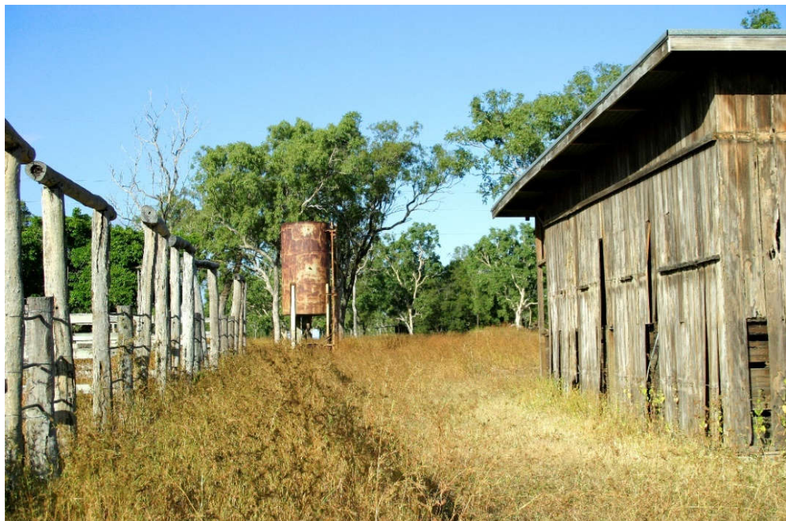
Old Building at Lakeland
