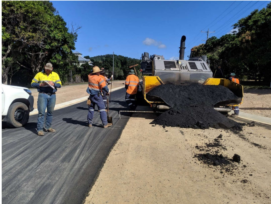
Cooktown - May Street Asphalt Sealing
